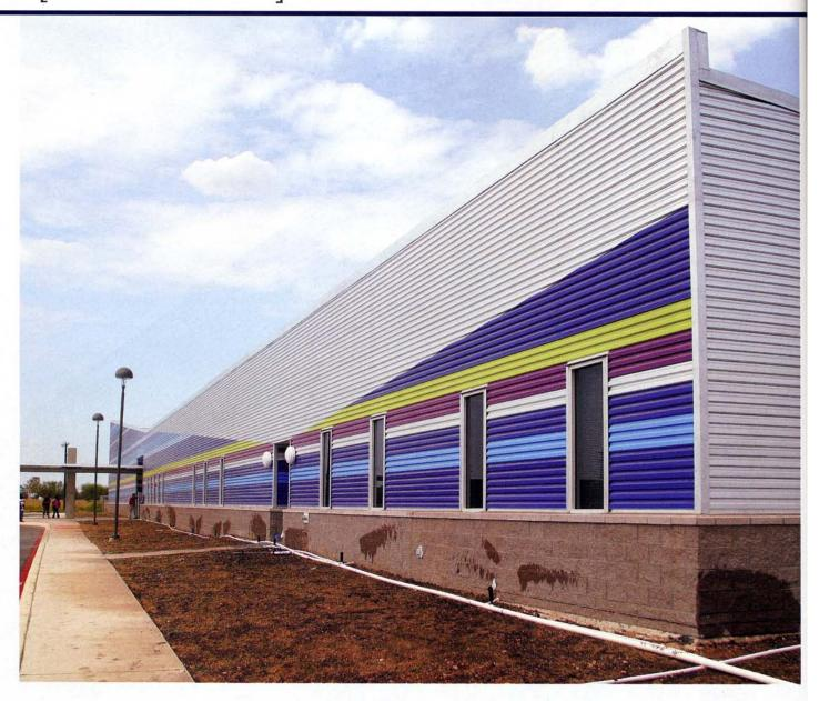
standard v-crimp panels. The area on the [Henry B. Gonzalez] convention center where we placed panels is where the new expansion will go. Because we used a metal panel system it will be easier to just take down the panels than destroying walls for the expansion," Sterner notes, adding that the convention center panels are finished in a custom color named "KMA blue" for the firm.
